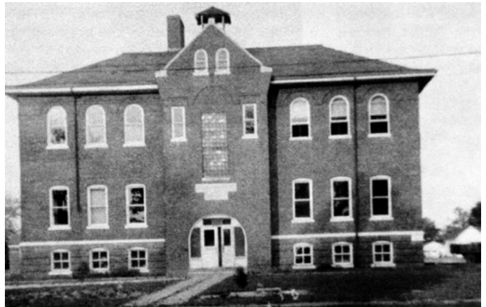
DIVERNON GRADE SCHOOL BEFORE BEING RAZED
